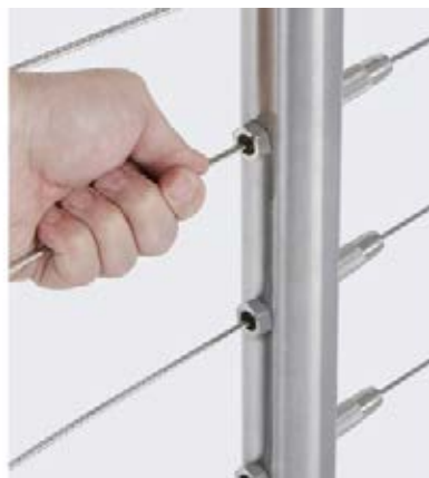
2. PULL CABLE THROUGH FITTING.
